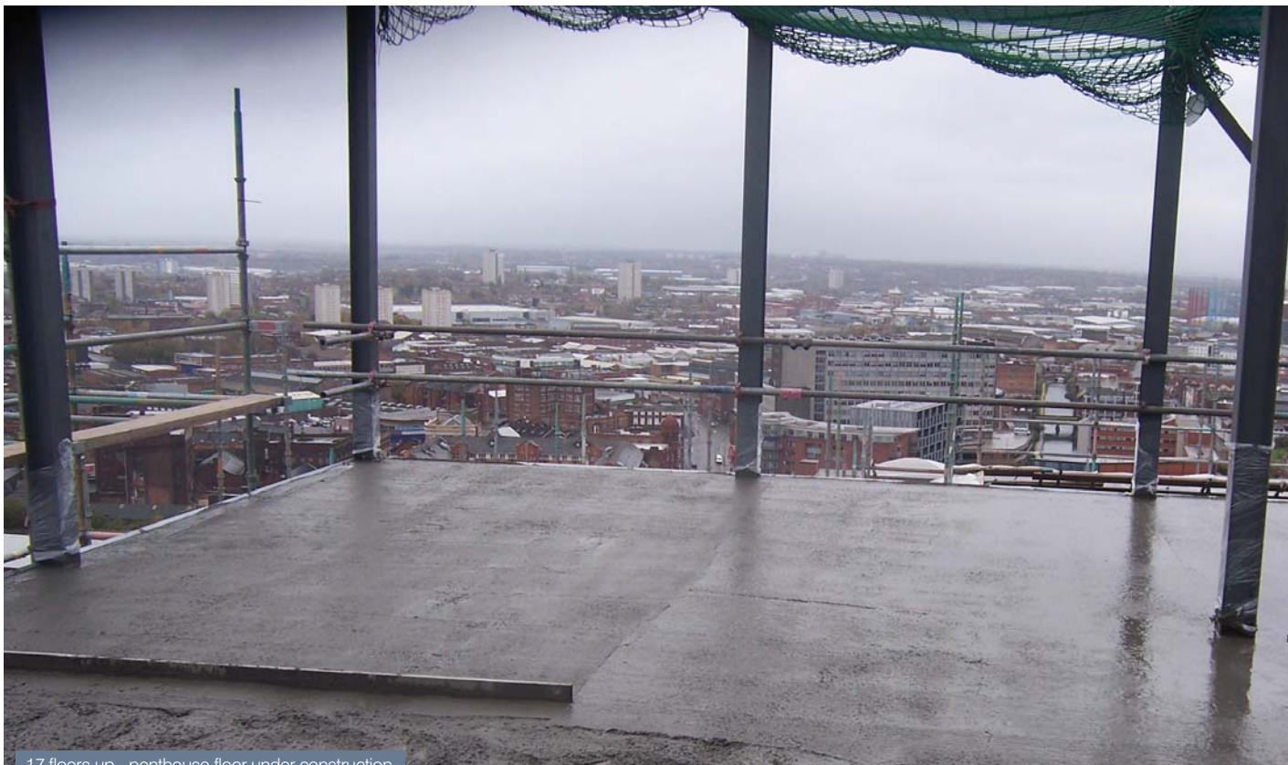
17 floors up - penthouse floor under construction
