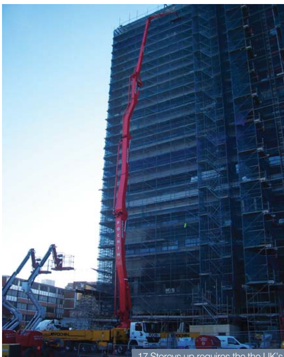
17 Storeys up requires the the UK's largest concrete pump
